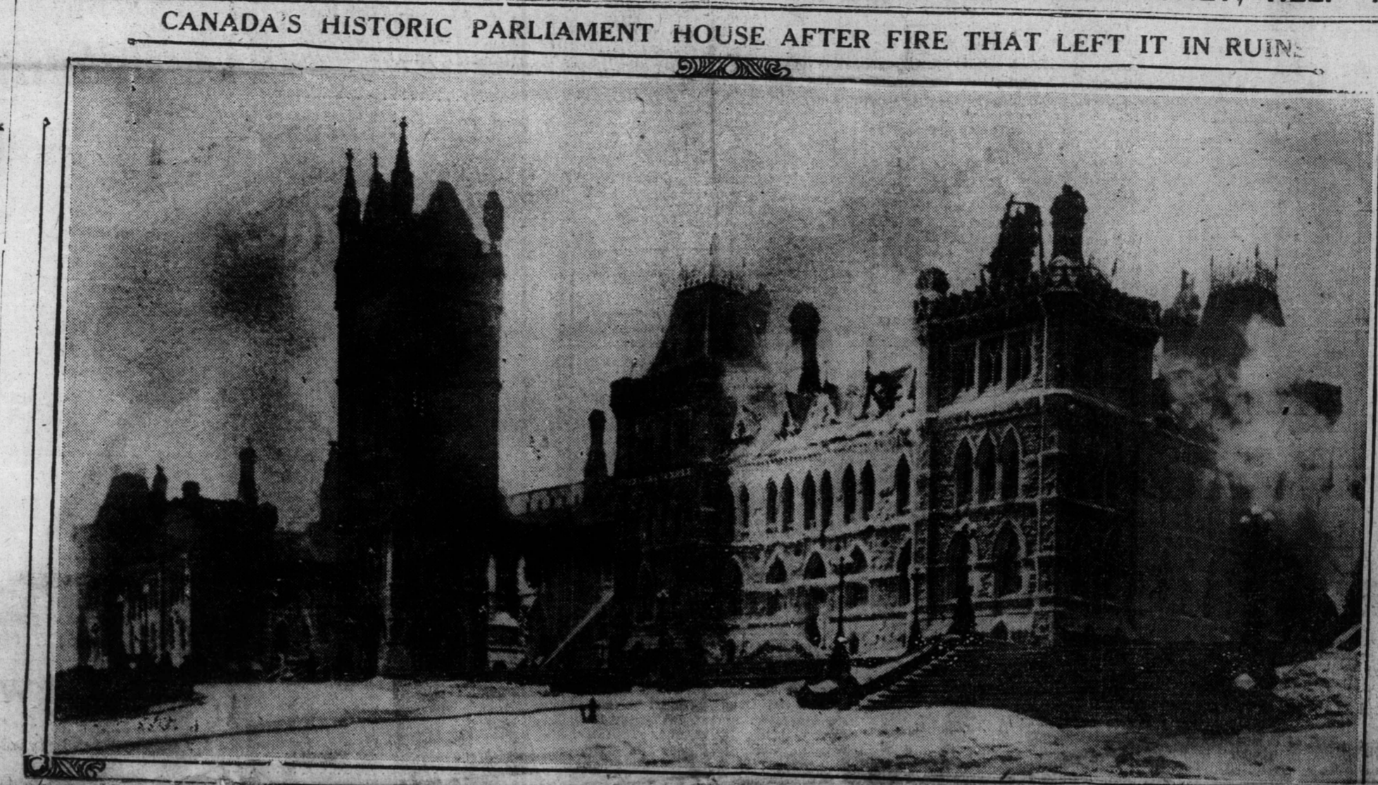
HERE IS SHOWN THE RUINS OF THE FAMOUS PARLIAMENT BUILDING AT OTTAWA, WHICH WAS DESTROYED BY FIRE, WHICH IS BELIEVED STARTED FROM AN EXPLOSION OF BOMB TERRORS SIMILAR TO THOSE PERPETRATED IN THE UNITED STATES.
