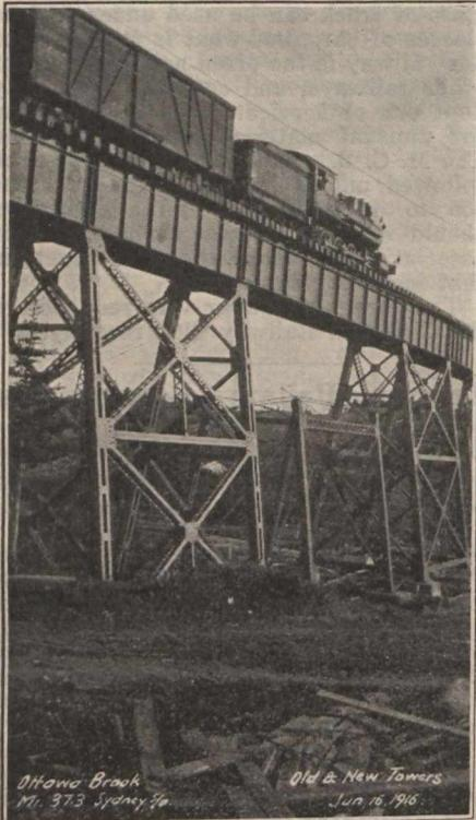
Ottawa Brook Steel Viaduct, showing new steel work in place, and old partly taken down.
