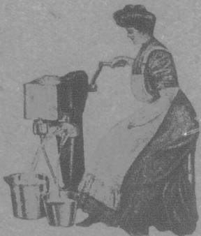
This is the Sharples Dairy Tubular. So simple and perfect in construction, that the medium sizes can be turned by one who is seated. Self oiling enclosed gears. Low, steady supply can.
