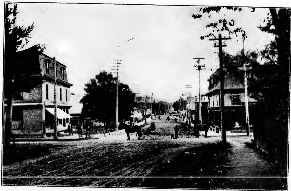
MAIN STREET, LOOKING EAST.
