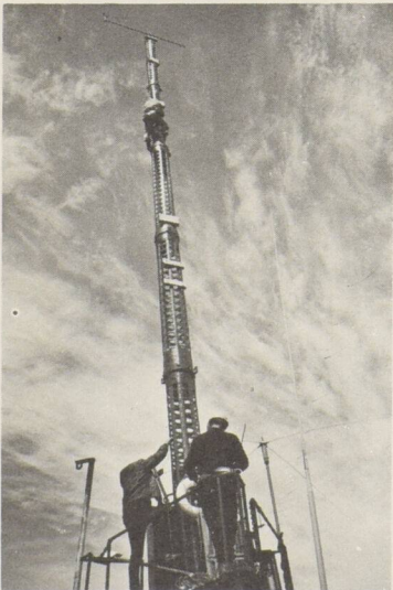
Meteorological sensors are attached at various levels on the fibre glass mast to measure wind direction, velocity and temperature.
