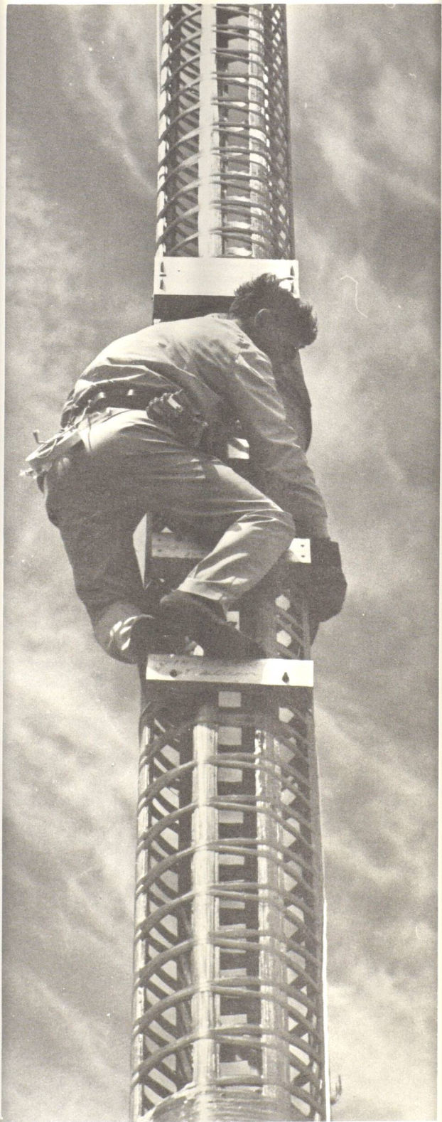
Stan Ozog, of the Meteorological Branch, securing sensor support to fibre glass mast.
