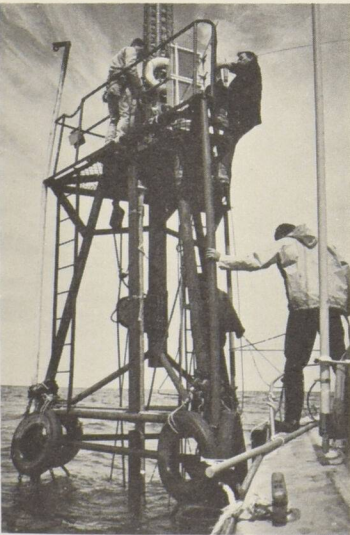
Meteorological Branch technicians ascend stable platform mast to service meteorological equipment.
