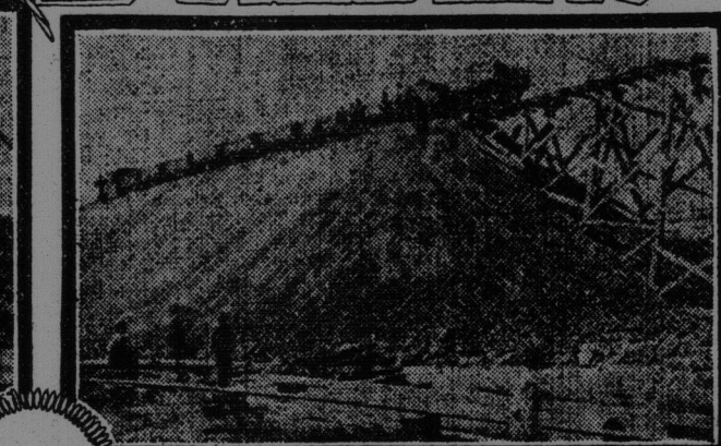
Building the Embankment or Approach
