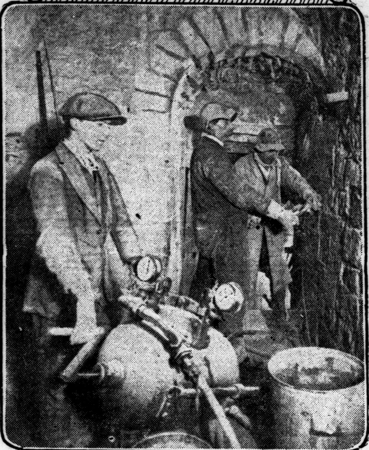
Dean Fry of Lincoln, is in Toronto to secure funds for the restoration of his cathedral. The pictures show the east side of the choir loft and a special machine for driving concrete by compressed air into the crevices in the stone work of the crumbling towers.
