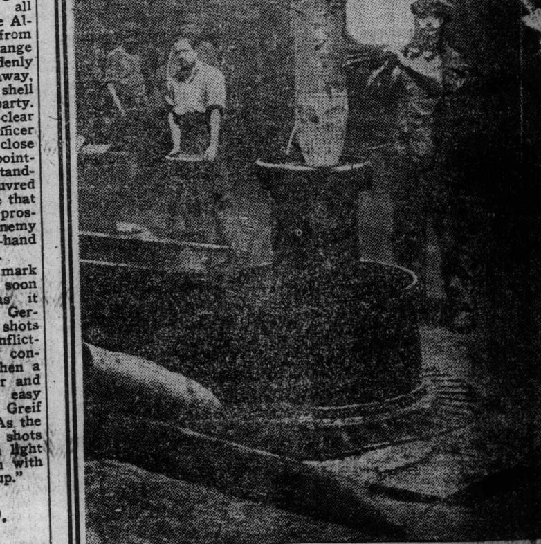
"LOWERING THE RED HOT SHELL INTO OIL"
