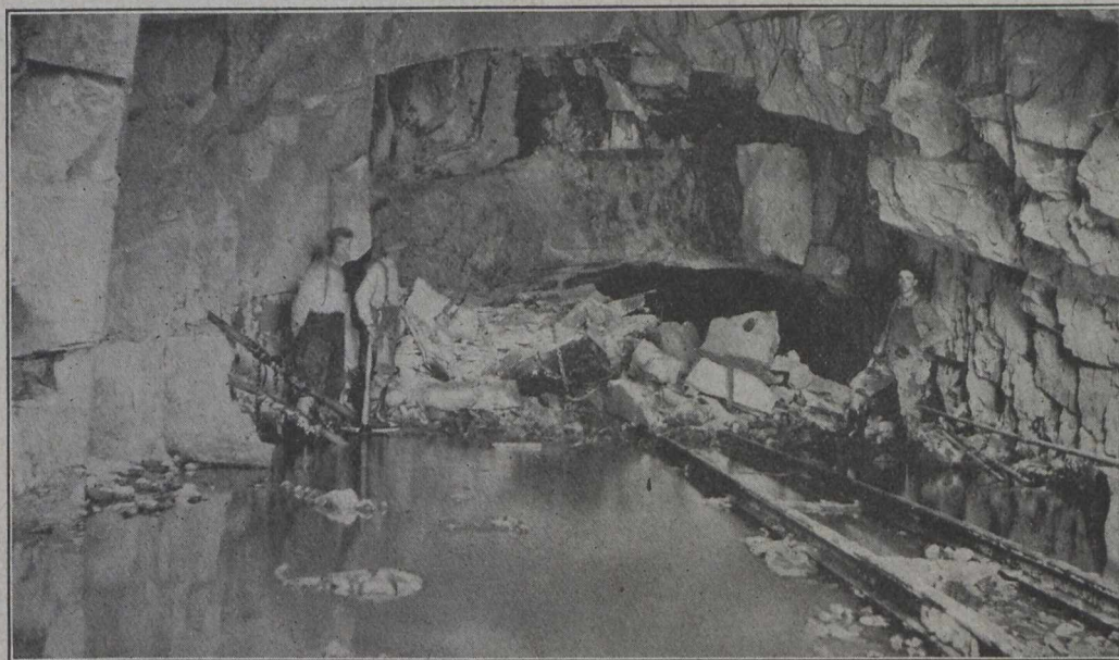
C.P.R. Water Tunnel at Keewatin
