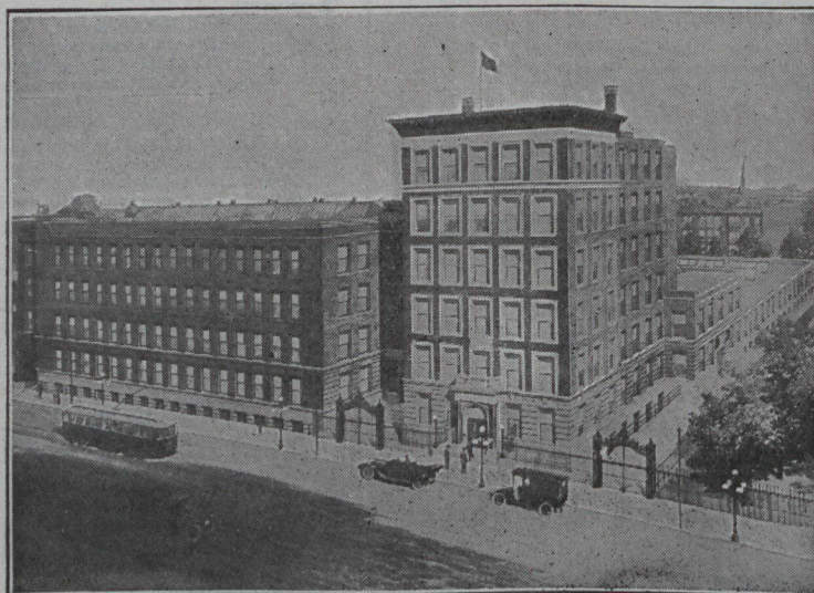
FIRE PROOF BUILDINGS
