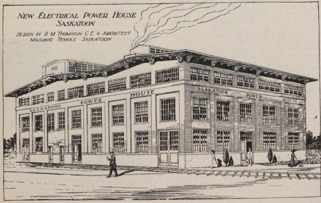
The construction is of steel, brick, and concrete, and is fireproof. The dimensions are 85 by 154 feet, and the walls are 42 feet high; the construction is of the most modern for
