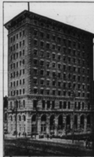
Union Bank Building, Winnipeg.
