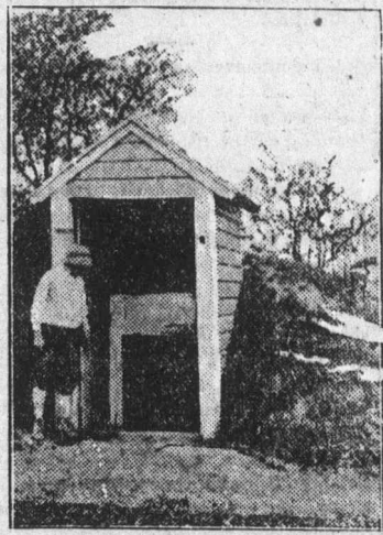
An Outdoor Storage Cellar, Built Partly Underground, for Storing Garden Vegetables. It is Built of Concrete. Except the Entrance, Which is Frame, and is Frostproof. Where the Cold It Not Severe Less Protection Than is Shown Here is Needed.
