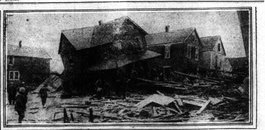
WRECKAGE OF FISHERMENS HOMES AT SEABRIGHT, N. J. Damage estimated at more than $1,000,000 was done recently by a northeast gale which swept the New Jersey coast. Sea Bright, N. J., where the gale attained a maximum velocity of ninety-eight miles, was almost devastated by the wind and the highest tide ever known there. Handsome cottages were swept into the sea, miles of board-walk and bulkheads destroyed and the streets torn up for yards inland.
