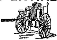
This machine is the most powerful fire fighter. It has two cylinders, 40 gallons capacity each. The combination of chemicals will not freeze, renders material with which it comes in contact non-inflammable, and ill not corrode when not in use. For full particulars, write to the Head Office of the Company at Kingston.
