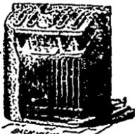
THE BACK of the JACKSON VENTILATING GRATE forms an air chamber in which outdoor air is heated. The latter can be sent to room above if desired.
