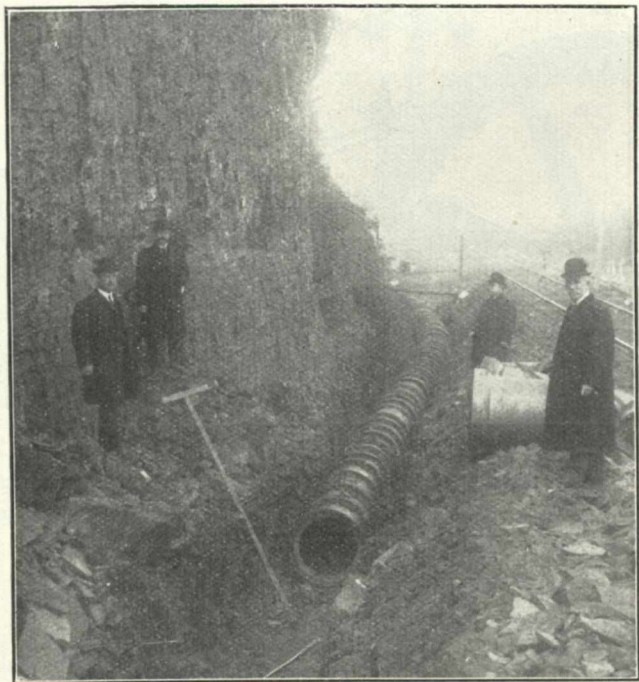
Pipe Line during construction.
