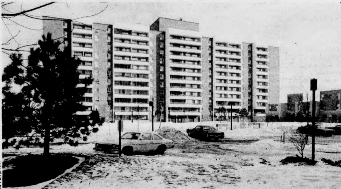
Part of Cadillac-Fairview's immense University City housing complex, just south of the York campus.
