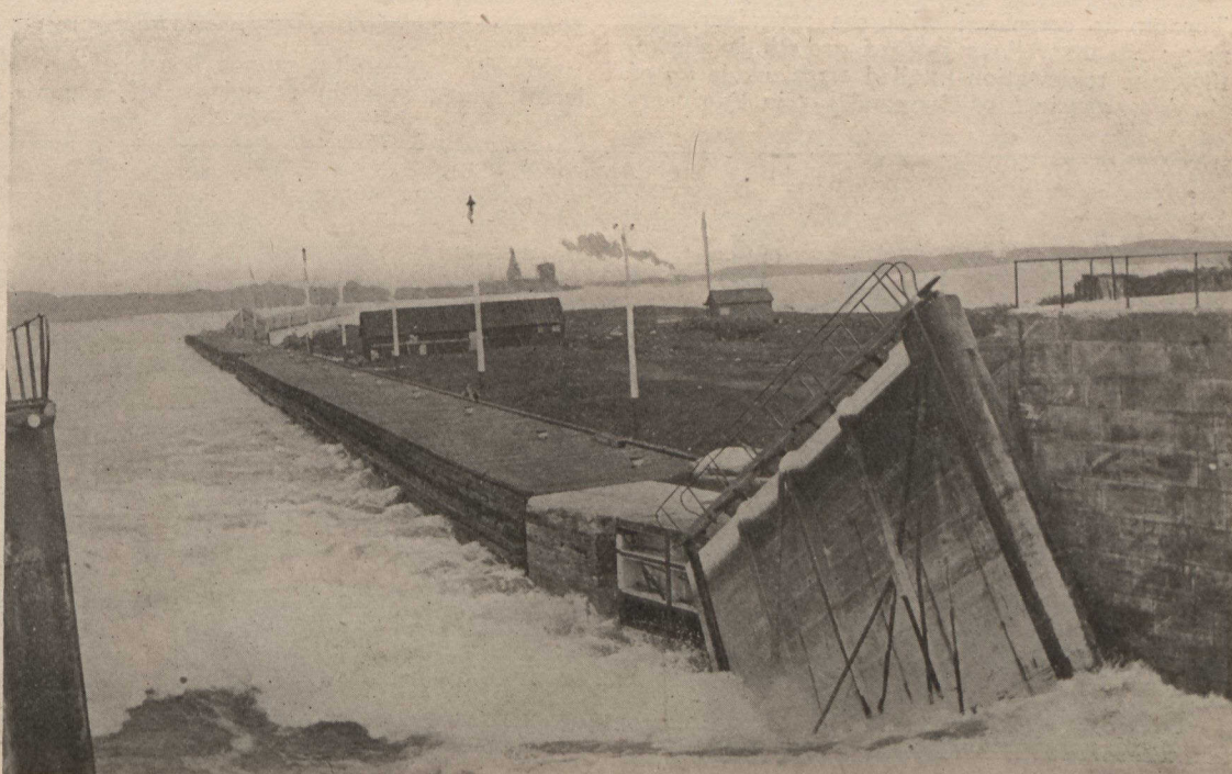
The Gates of the Sault Canal, broken last week, causing damage estimated at a quarter of a million dollars.
