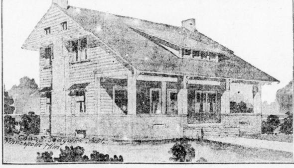
HERB the lot will admit of it, a wide front is always the best. This cottage is 38 ft. in width and 32 ft. in ft. in width and 32 ft. in depth over the front piazza, which is 10 ft. in width. The plan is well suited to an east frontage, bringing the large living room on the south side and also to the east. It is estimated to build this cottage for \$3,500 to \$4,300 exclusive of heating and plumbing. It is of well constructed frame, covered with wide Colonia
