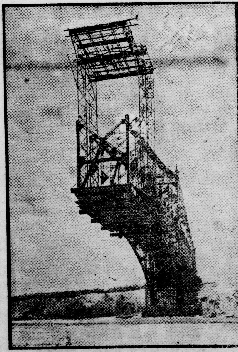
VIEW OF COLLAPSED SECTION OF QUEBEC BRIDGE AS SEEN FROM THE RIVER.
