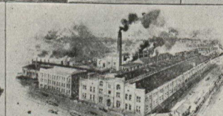
NEW FACTORY BUILT IN 1890 SINCE THEN THE FOLLOWING EXTENSIONS HAVE BEEN MADE MACHINE SHOP 100' x 100' NOW 220' x 80' WITH CORRESPONDING BOILER SHOP 100' x 100' NOW 220' x 80' INCREASE BLACKSMITH SHOP 40' x 100' NOW 100' x 90' IN EQUIPMENT.
