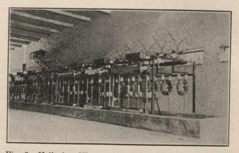
Fig. 8.-Vallorbe: Water Resistance Lightning Arrester.
