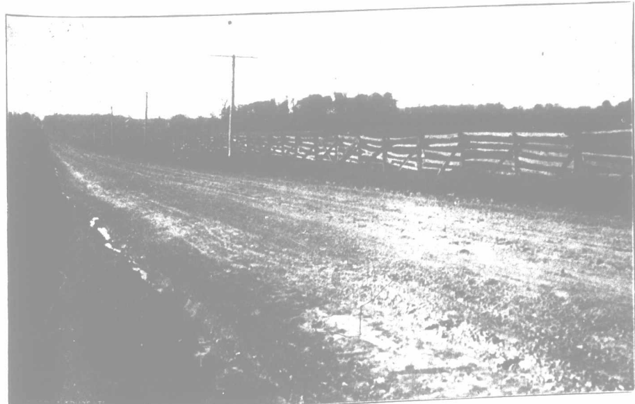
Cherry Avenue—a mile of splendid clay and sand road dragged the third year by W. J. Stattenhouse, whose farm at the north end of the beat is bordered by rows of cherry trees. This road has been graded from a rut condition with the split-log drag, and maintained like a turnpike. Also graded last year.
