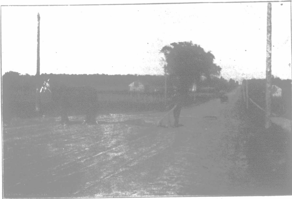
Half-mile on the Fly road dragged by J. M. Wismer. This road was too wide and was in many places ridged in the center, but flat between center and shoulders. Has been narrowed from 36 to 30 feet, shaped up nicely and kept smooth, all with the King ditcher and the split-log drag. Note the lift-lever on drag, devised by Mr. Wismer.
