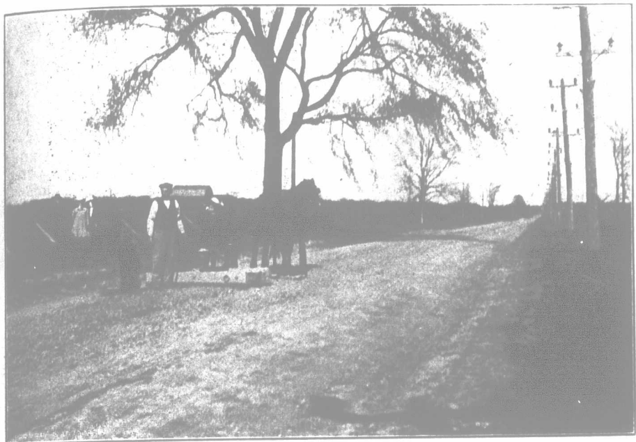
Road being dragged for the third season by D. H. Moyer, who has had his beat graded by the township on condition that he was to maintain it without charge for five years. Note that the drag is being run backwards to smooth down and spread the small ridge of loose earth left at the last time across.
