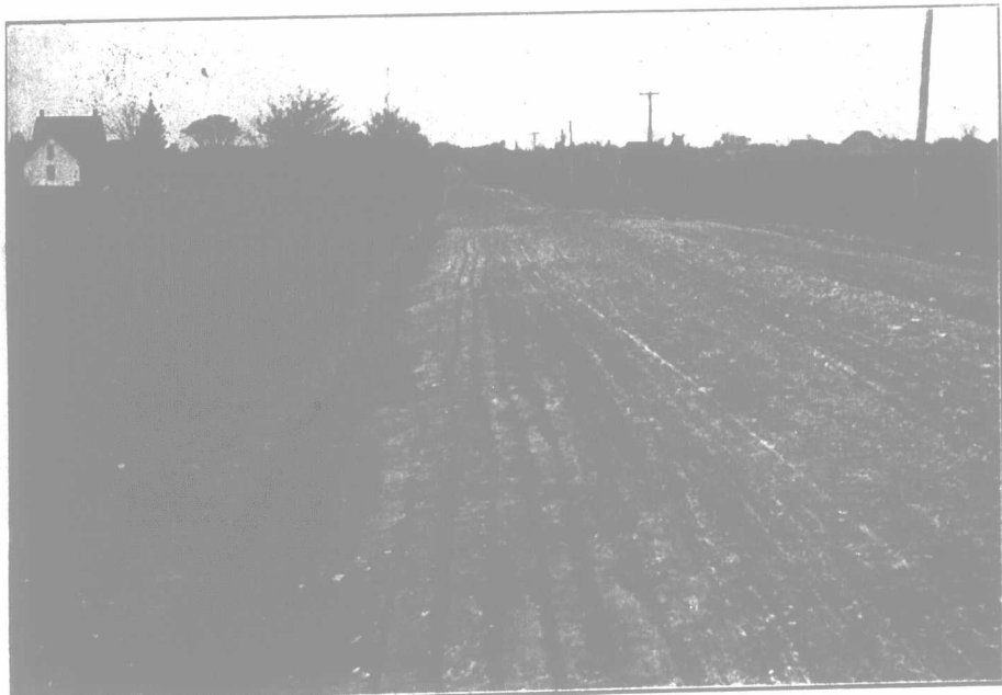
A road in the making. Five-eighths of a mile that has been greatly improved by Angus Stewart. Disk marks show on side where the loosened earth has been drawn to the center with the drag.
