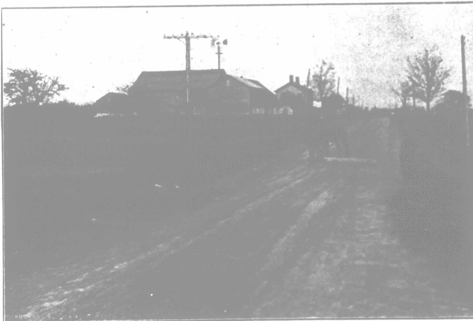
Half-mile of good clay road dragged by Frank Love. The camera has exaggerated the slight imperfections along the track.
