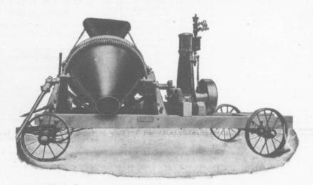
The above illustration shows one style of Smith Mixer. This machine is fitted with niggerhead for hoisting purposes. Space is left on the truck behind the engine for mounting boiler.
