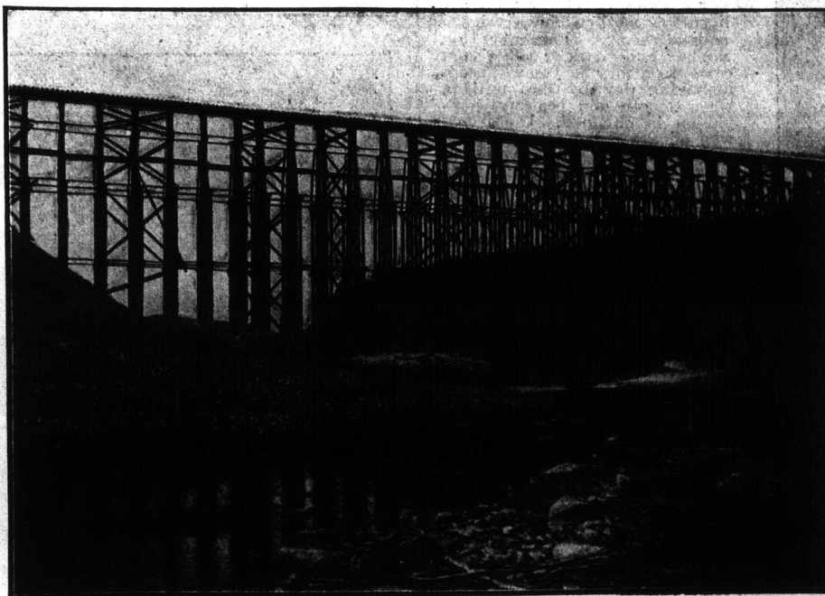
Trestle near Wolf Creek, Alta, G.T.P.
