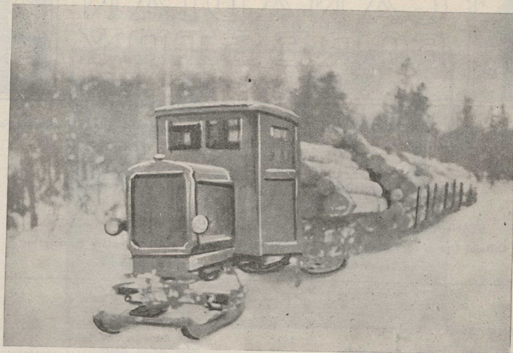
LINN LOGGING TRACTOR ON OPERATION OF ST. MAURICE PAPER CO., AT ST. DONAT DE MONTCALM, QUE.
