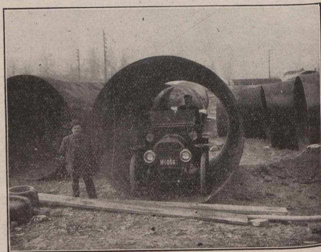
Kensico Siphon—15 ft. Section of 9 ft. 9 in. x 7-16. in. Steel Pipe. Size shown by automobile.
