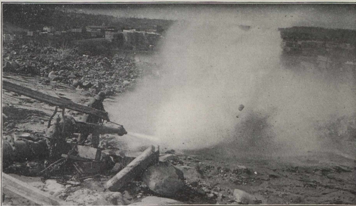
Cleaning Rock Surface, Nipissing Mine
