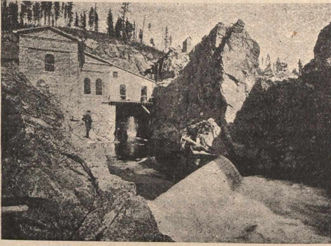
Figure 3.—Rear View of Power House Showing Draught-Tube and Tail Race.
