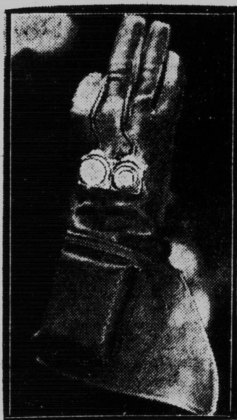
A new device for motorists. This gauntlet, bearing in it an electric torch, is for use in turning street corners at night when the driver's signal might not be seen by the car behind.
