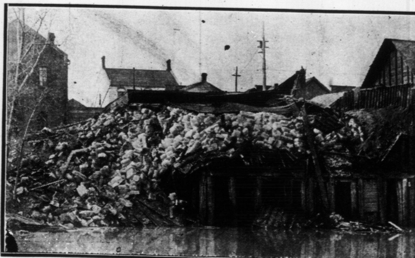
DESTRUCTION OF THE FLAVELLE COLD STORAGE PLANT, CHATHAM, ONT., APRIL 22. Wrecked building on the River Thames, showing many tons of ice, the weight of which caused the building to collapse. Jam under Third-street Bridge, caused by the debris of wrecked building lodging between the pillars.
