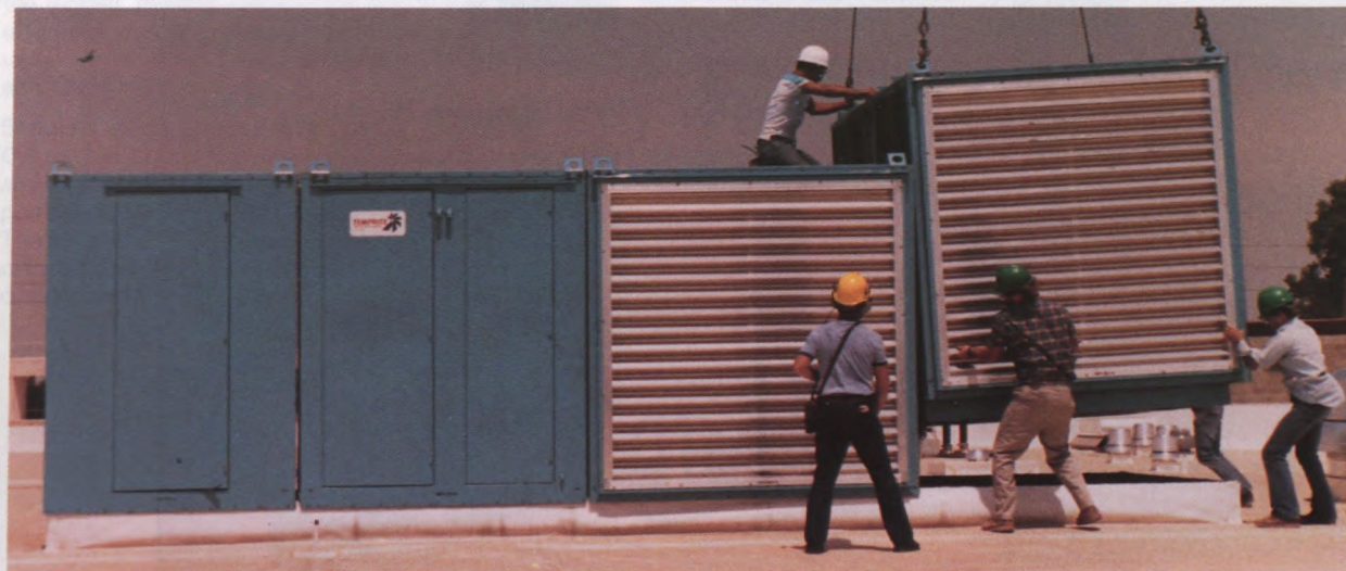
The HRX 25 is a 20 000 SCFM heat-recovery unit with a direct-fired gas burner; the heat exchanger is an aluminum plate type design that recovers 68 per cent of the exhaust air energy for preheating the incoming fresh air.
