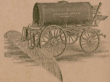
AUSTIN STEEL STREET SPRINKLER
