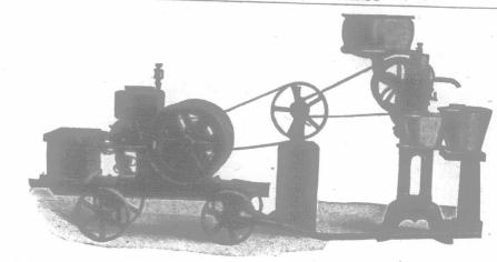
This MONARCH 1½ h.-p. Engine attached to our Intermediate Friction Clutch Pulley solves one of the problems for hired help. No counter shaft needed with this attachment.
