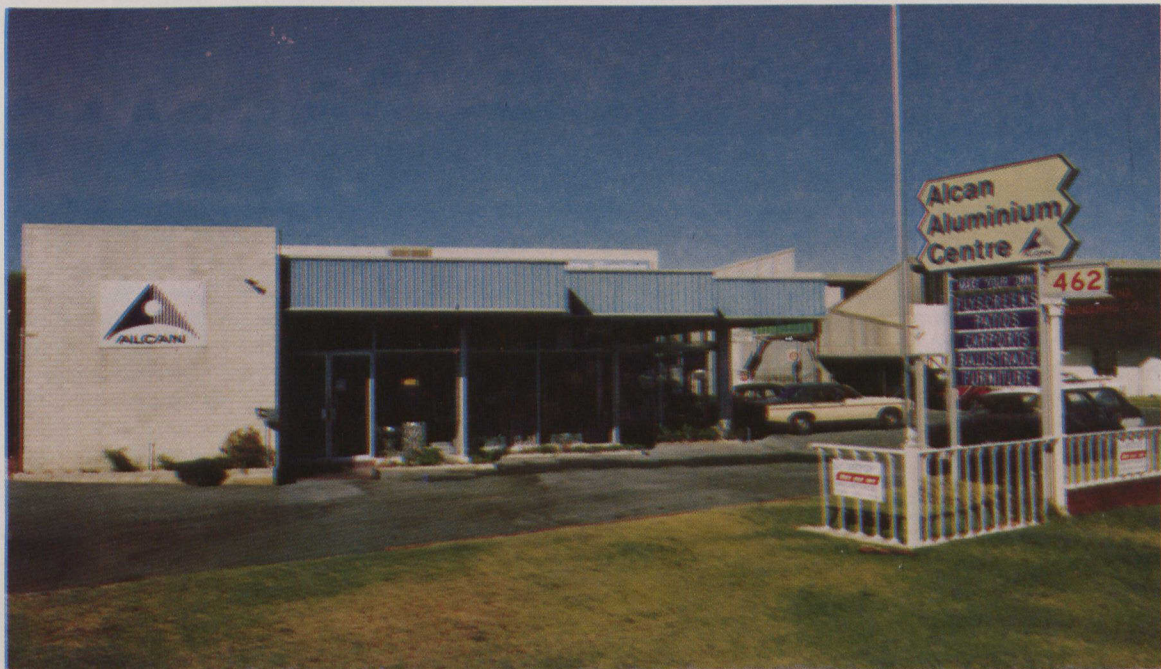
Alcan Aluminium Limited's Osborne Park aluminium centre.
