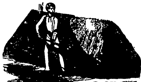
Fig. 2.—Covering Heap with Earth.
