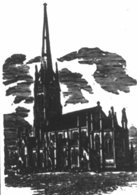
St. James' Cathedral, King St., Toronto, contains 500,000 cubic feet of space and is successfully heated with four of our Economy Heaters.
