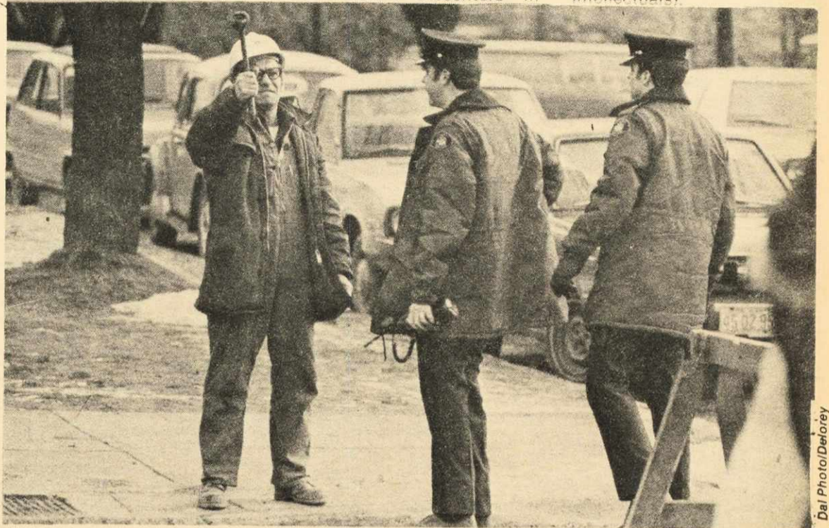
Construction worker on LeMarchant Street complains vehemently about picketers moving his barricade to University Avenue.
