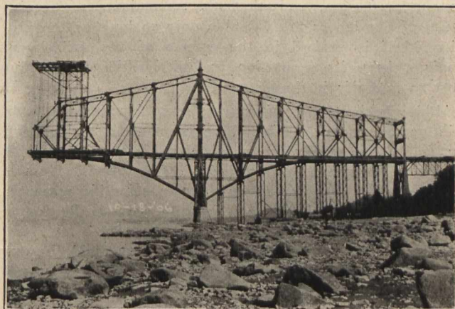
Quebec Bridge.—South Cantilever Arm.
