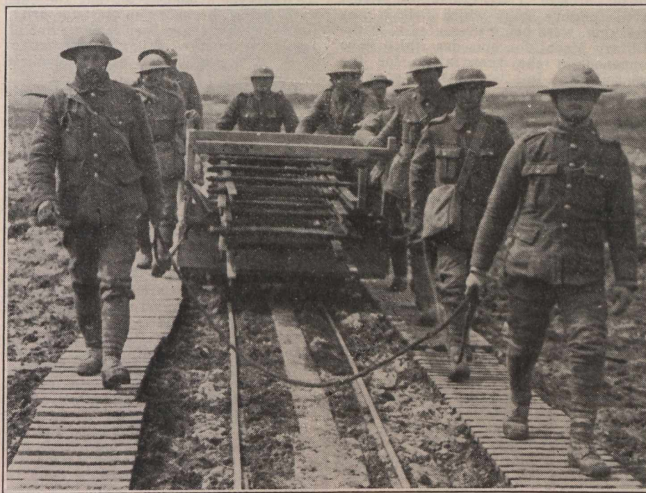
Light railway laid over captured ground on the British Western Front Official photograph issued on behalf of The Press Bureau. Crown copyright reserved. Loaned by C.P.R.
