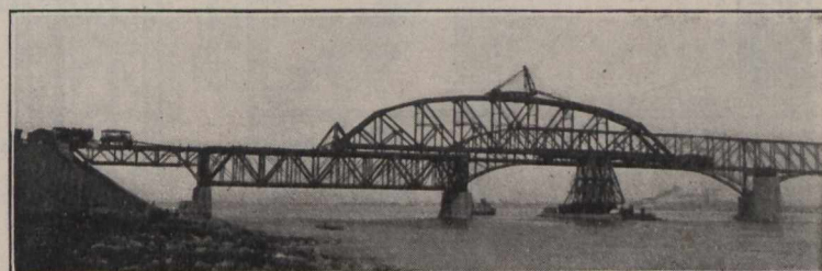
Down Stream Span 13-14 Being Launched, Showing the Lidgerwood Engine and Sliding Buggy.
