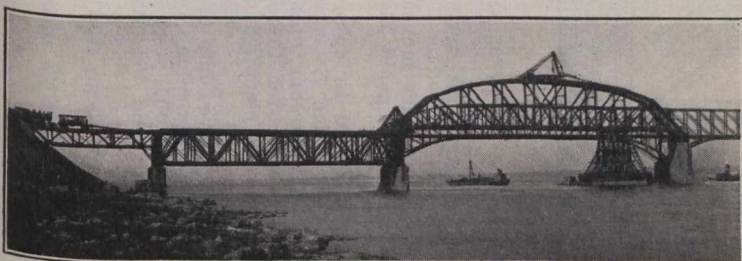
Down Stream Span 13-14 During Launching. Span Has Just Been Landed.
