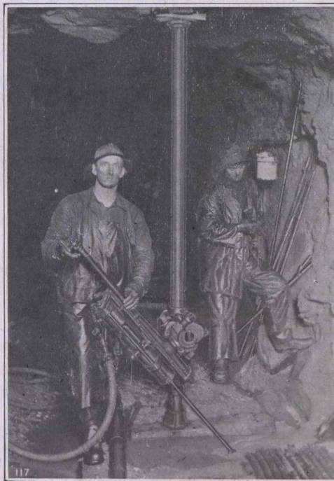
One of the Denver "Dreadnaught" Drills in the Rogers Pass Tunnel, Glacier, B.C.
