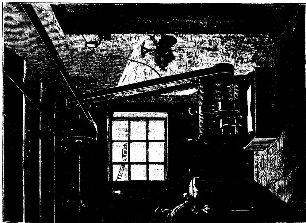
FIG. 6.—INSTALLATION AT MIESBACH.
