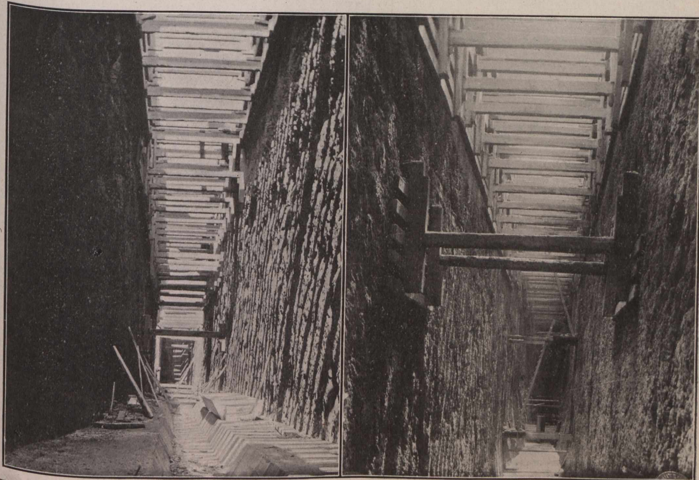
Fig. 1.—Trenching Methods, Delph Reservoir, Eng.—(Right) Rock Section Trench Bottom Ready for Concrete. (Left) Concrete Completed in Trench Bottom.
