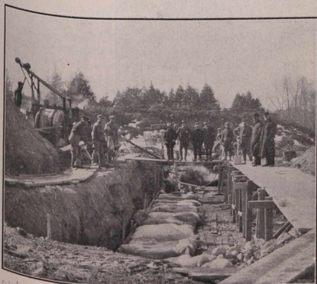
Fig. 7. Straw Ticks Over Concrete.
