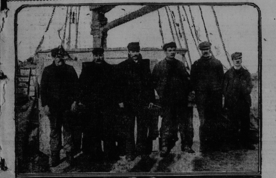
Part of Roosevelt crew on main deck of vessel. Second and third men from the left are Geo. Wardwell, Chief Engineer, and Thos. Gushue, the mate.
