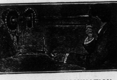
Lighthouse for the roads. An acetylene lamp, erected at Sidcup, England, flashes six times a minute and warns of dangerous crossings.
