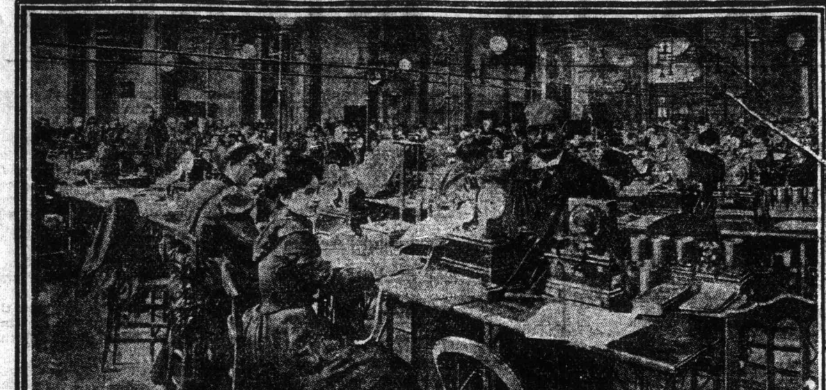
MAIN OPERATING ROOM OF THE PARIS CENTRAL TELEPHONE EXCHANGE.
