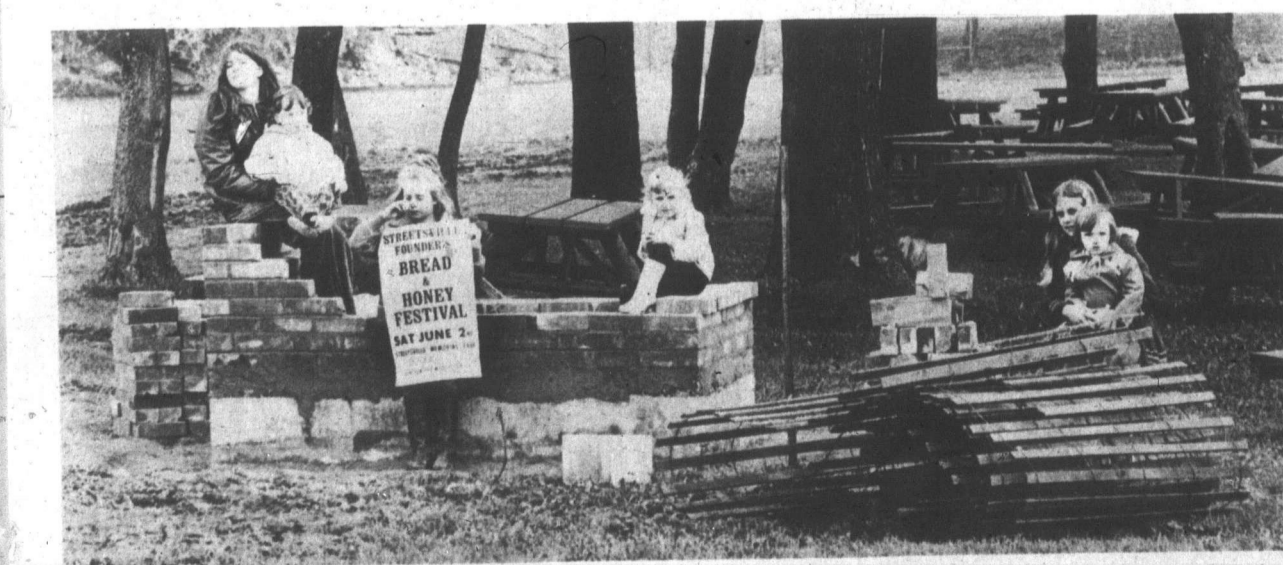
Oven is being built for bread-baking contest.
